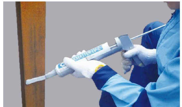
5) Apply LEAKMASTER LV-Z continuously without a break to the place to be sealed
